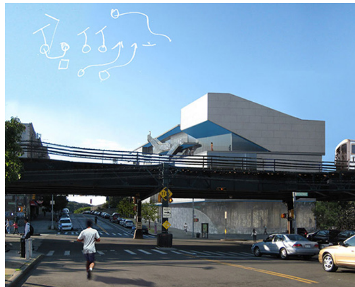
Campbell Sports Center at Columbia University, New York, City. © Steven Holl. Courtesy Steven Holl Architects.
