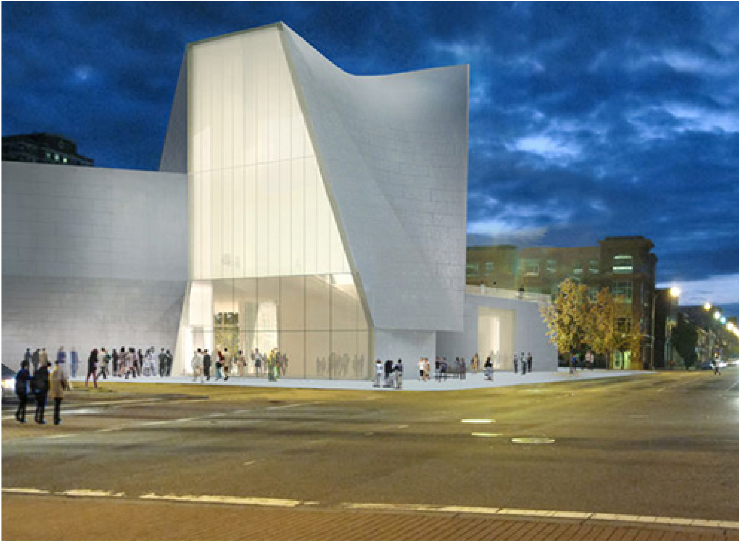
Institute For Contemporary Art, Virginia Commonwealth University, Richmond, Virginia © Steven Holl. Courtesy Steven Holl Architects.
